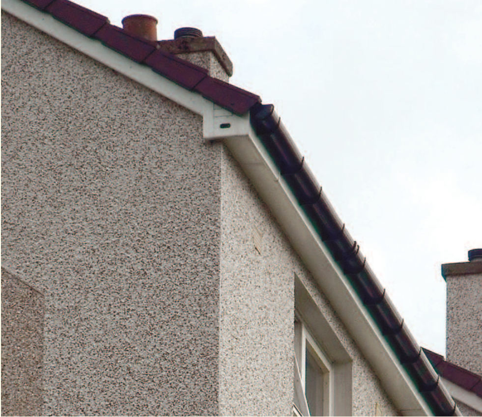
Plate 306. A hole cut in to the PVC soffit on the gable now provides a better design. © Clare Darlaston
